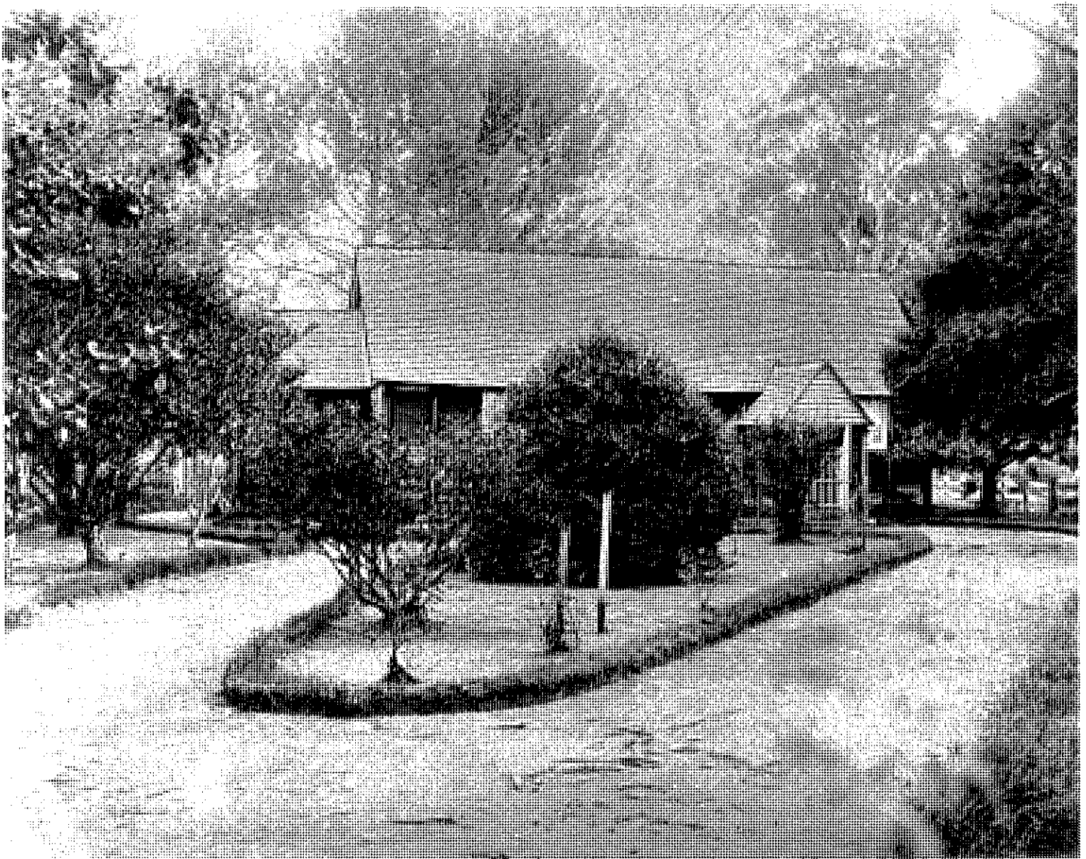
Fig. 42 : The first St. Anne's Anglican Church at Gresford, replaced in 1898 by the present brick St. Anne's. The modest scale and slab construction is typical of the early stage of church-building in the Shire. (Mitchell Library).
