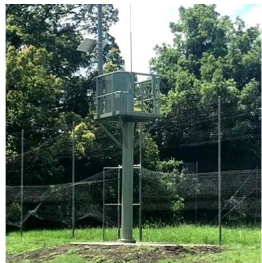
Flood gauge in Alison Court, Dungog
