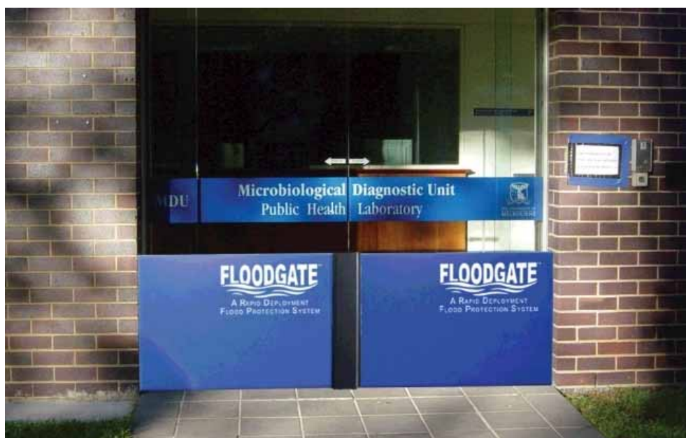
Figure 7-20 Temporary Floodgate Flood Barrier (source: http://www.hydroresponse.com/floodgate.htm )
