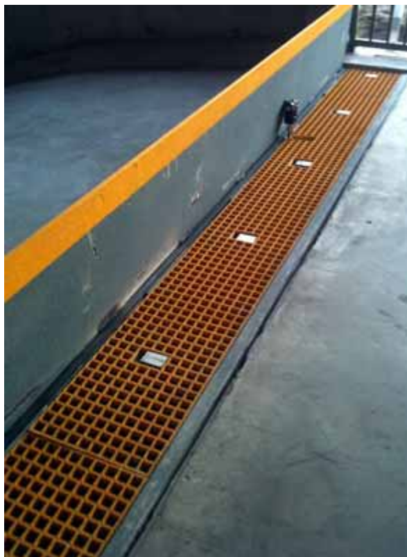
Figure 7-19 Permanent Automatic 'Flip up' Flood Barrier (source: http://www.spec-net.com.au/press/0212/flo_150212.htm )
