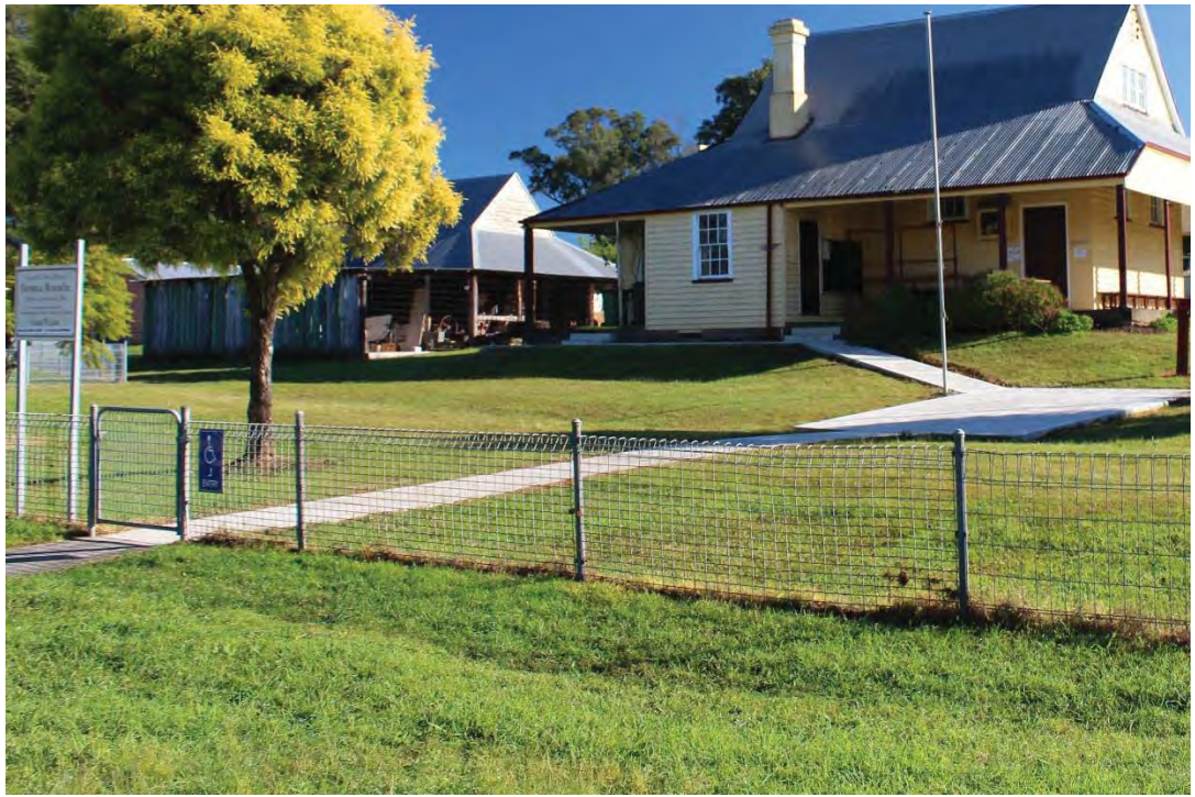
Figure 61: View of the weld mesh fence which defines the southern boundary of the Clarence Town Courthouse site
