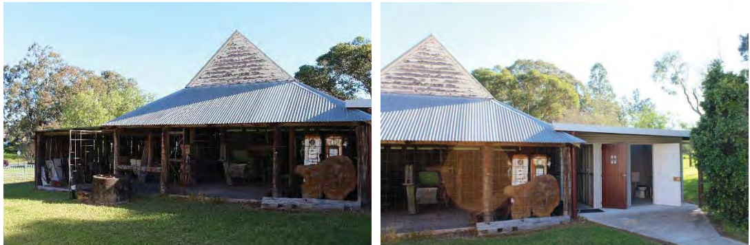
Figure 44: Views of western elevation of the Outbuilding, with the open shed structure containing museum pieces to the left and the northern addition visible to the right.
