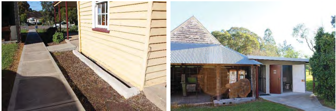
Figure 59: View of the pathway which leads from the boundary of Grey Street, to the Courthouse (left) and onto the bathrooms located in the northern portion of the Outbuilding (right).
