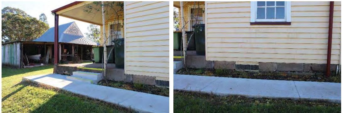
Figure 24: South-western verandah (left) and sandstone footings and ventilation grates visible on the southern elevation (right)
