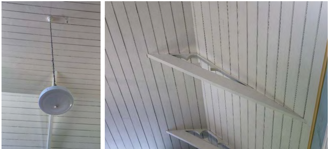
Figure 29: Detailed view of the suspended light fixtures (left) and exposed purlins and decorative timber brackets in the Court Room (right)
