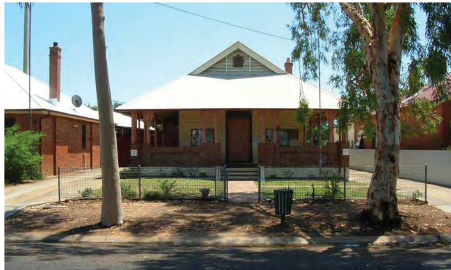
Figure 122: Gilgandra Courthouse viewed from Myrtle Street (Source: SHR form for Gilgandra Courthouse, http://www.environment.nsw.gov.au/heritageapp/HeritageItemImage.aspx?ID=3080057#ad-image-0 )
