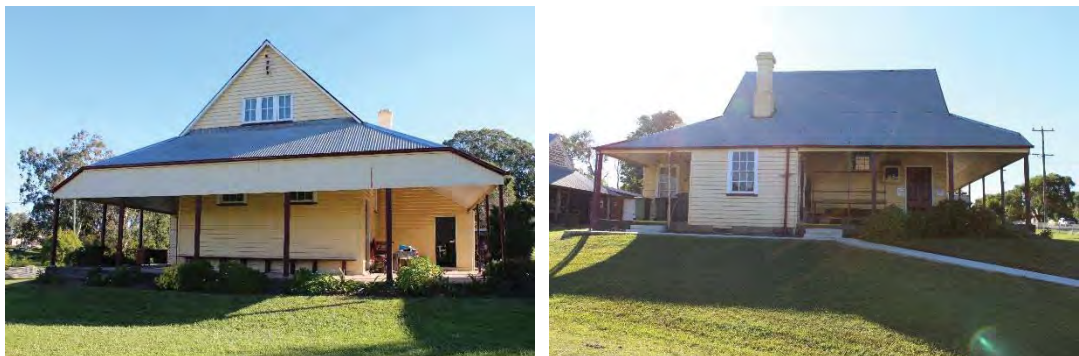
Figure 21: Eastern elevation (left) and southern elevation (right) of the Clarence Town Courthouse
