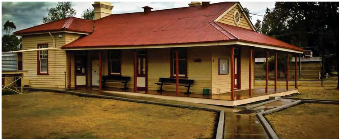
Figure 121: Boggabilla Courthouse viewed from Merriwa Street (Source: Rapid Construction, http://www.rapidconstruction.com.au/projects/boggabilla-court-house-refurbishment/ )
