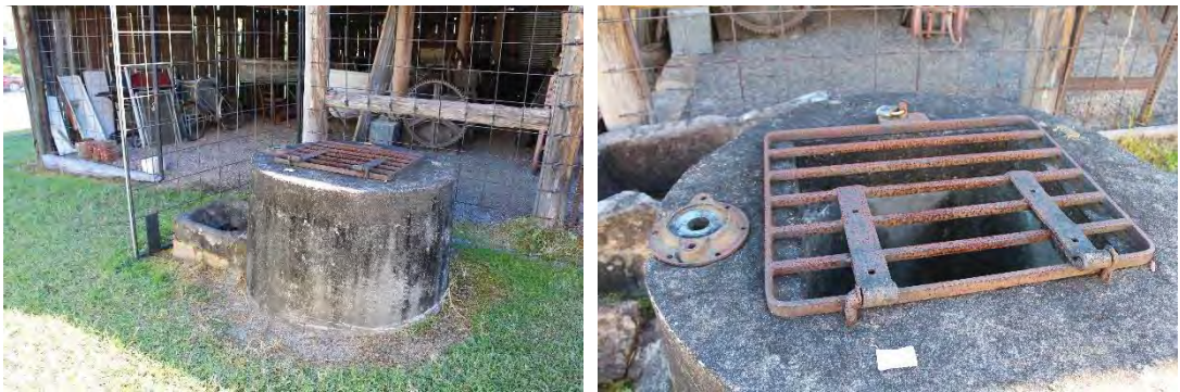
Figure 51: View of the well which is located directly to the east of the Outbuilding (left) and a detailed view of the well with existing grill and location of where the hand pump, now missing, was once positioned (right)
