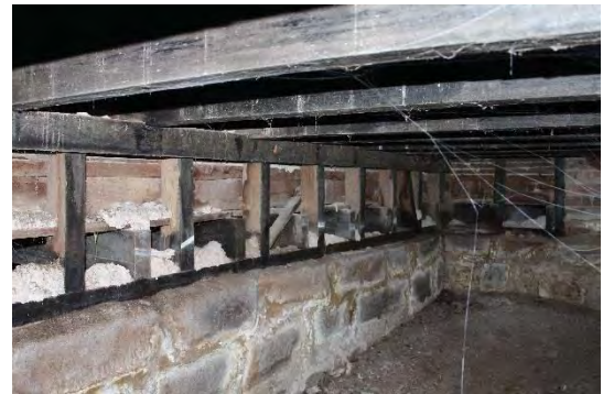
Figure 31: Base platform of the magistrate's bench in the Court Room (left) and view underneath the platform of the magistrate's bench, revealing the sandstone footings (right)
