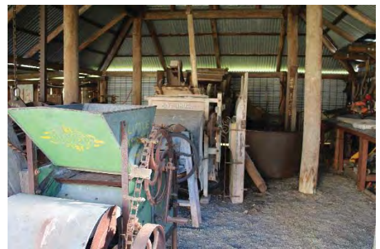
Figure 47: View of the interior of the Dutch gable roof of the Outbuilding, with timber posts, beams and rafters, the corrugated metal cladding on the roof being laid directly onto the rafters (left) and view of the middle section of the Outbuilding directly under the apex of the Dutch gable form roof (right).
