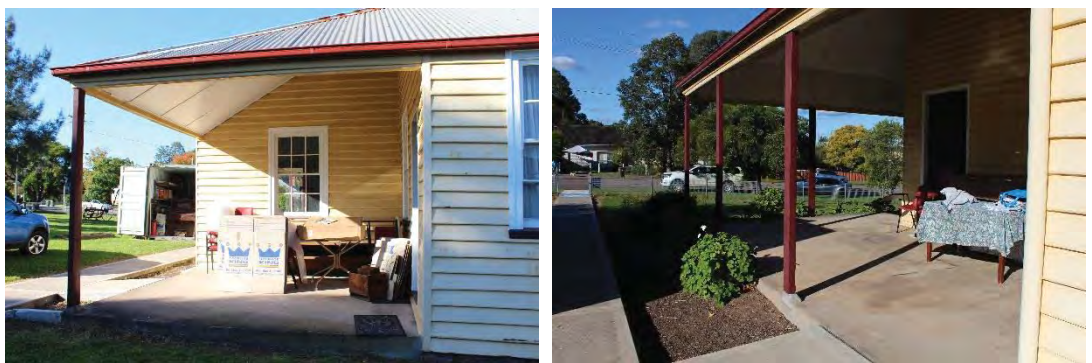
Figure 25: North-western verandah (left) and northern portion of wrap-around verandah (right)
