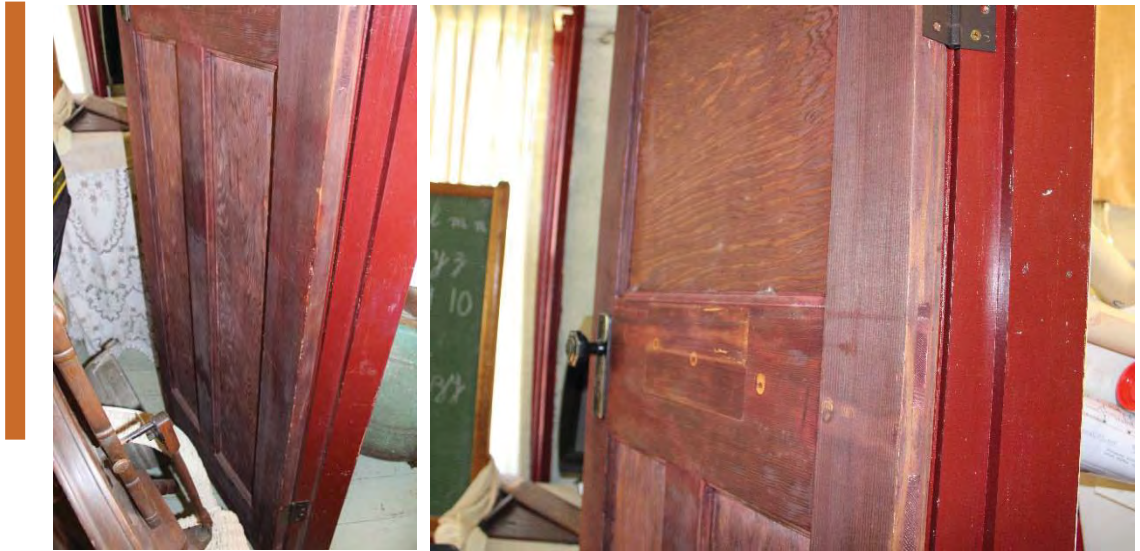
Figure 41: Views on the base (left) and top (right) of three-panels mid-20th century door located in the dividing wall of the Store Room.
