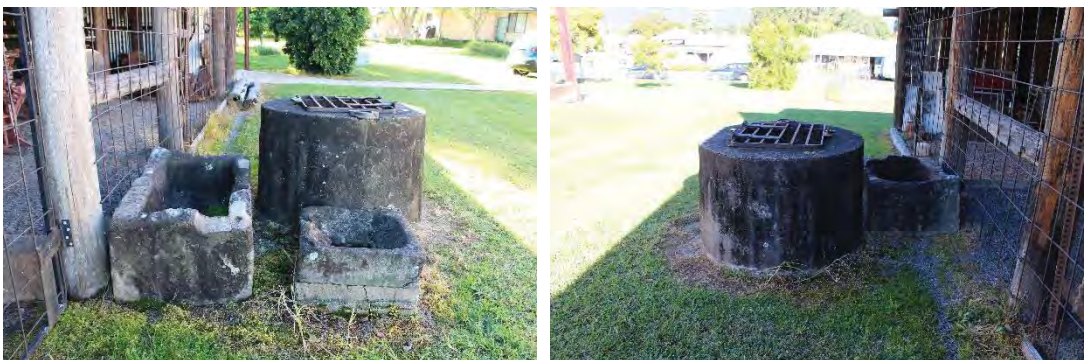
Figure 52: View of the well, small trough, formerly located under the hand pump and horse trough from the south (left) and view of the well and horse trough from the north (right)
