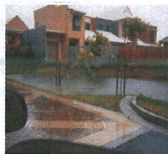
DETENTION BASIN EXAMPLES MORE INFORMATION ON DETENTION BASINS IS AVAILABLE IN THE TOWN CREEK PLAN OF MANAGEMENT - 'APPENDIX B'
