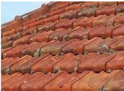
Existing Roofing (RF.EX.01) Terracotta/Clay Tile
